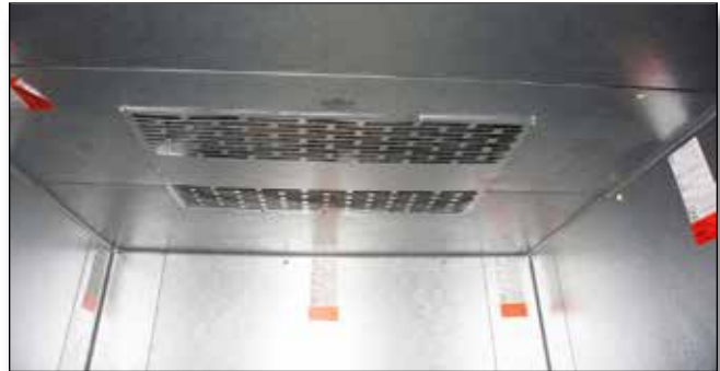
The Capsule Pak evaporator grille mounts flush in a standard 4" thick ceiling panel allowing maximum storage space inside the walk-in.
