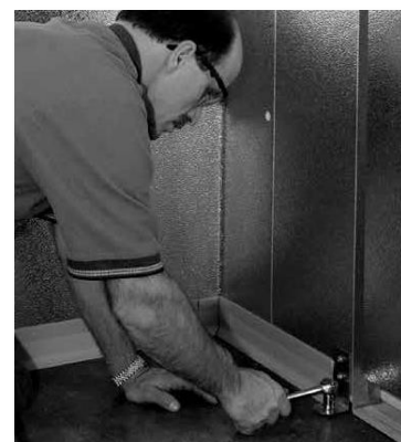
Attach slam brace with fastener provided
