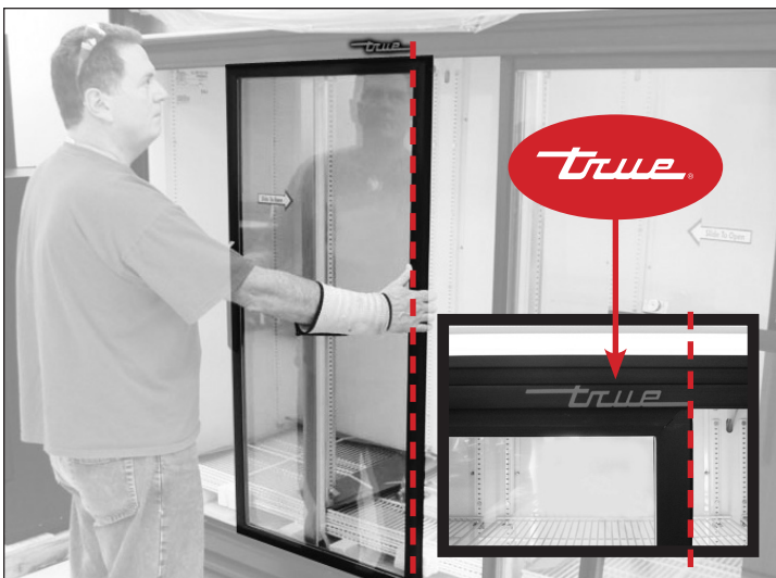
Fig. 6. Align the right edge of the left door with the right edge of the TRUE logo.
