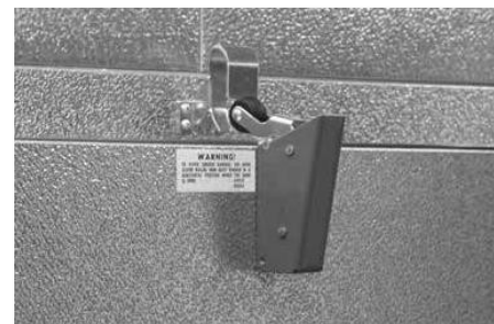
Roller Too High
