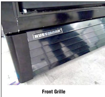
Lift up, and pull off the grille.
