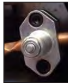
refrigeration line tapping valve
